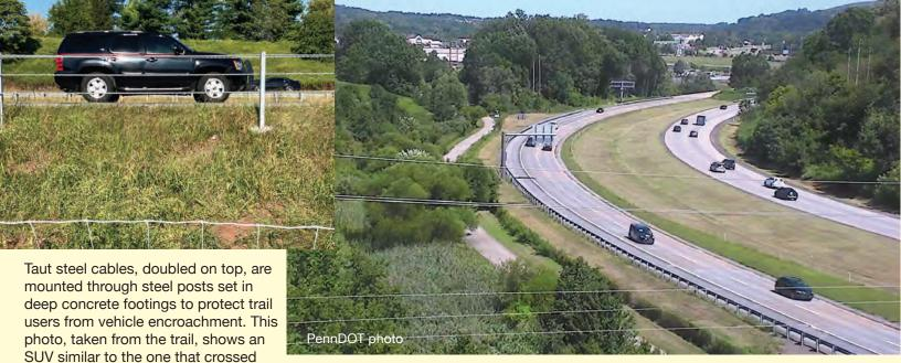
The heavily used Schuylkill River Trail runs parallel to and below the grade of Route 422. Last summer, before the safety improvements, a tractor-trailer left the westbound lanes (right in uprooted, the cables would ensnare the photo) crossed the median, and hit a eastbound SUV so hard it ended up crossing the trail.
